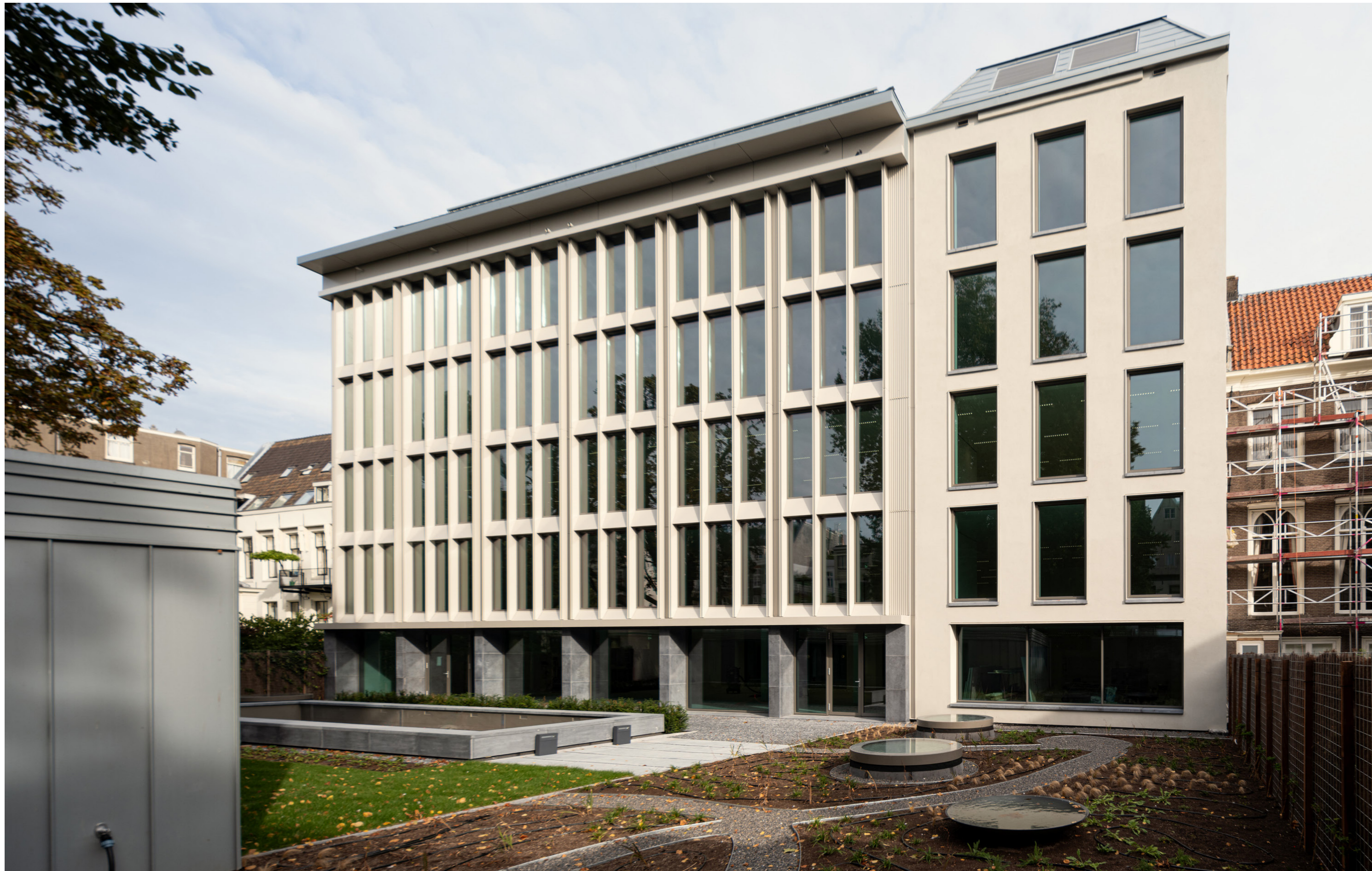
Vista Exterior General
